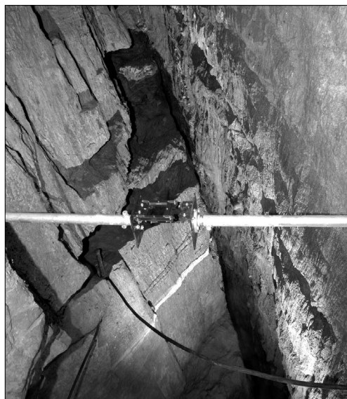
Fig. 5. TM71 gauge (extensometer) installed across the WSW – ENE trending passage. Photo: P. Blaženín
