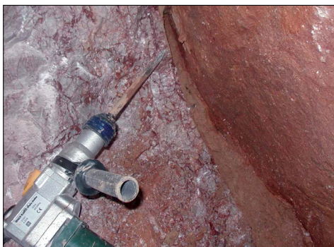
Obr. 2. Porucha vyplnená hlinou, na ktorej sa razil nový vchod. Foto: Z. Hochmuth Fig. 2. Dislocation filled by the clay, where was digged the new entrance along. Photo: Z. Hochmuth
