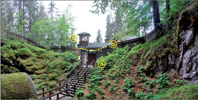
Fig. 1. Entrance Collapse of Dobšinská Ice Cave – view from SE side – present state: a) artificial ditch in the Collapse edge; b) position of the fence edge (dashed line) before modifications; c) decorative turret with openings covered by a Plexiglas plate. Photo: T. Sawiński, July 2012
